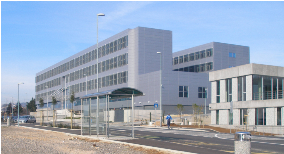
Figure 3: Faculty of Civil Engineering, University of Rijeka
